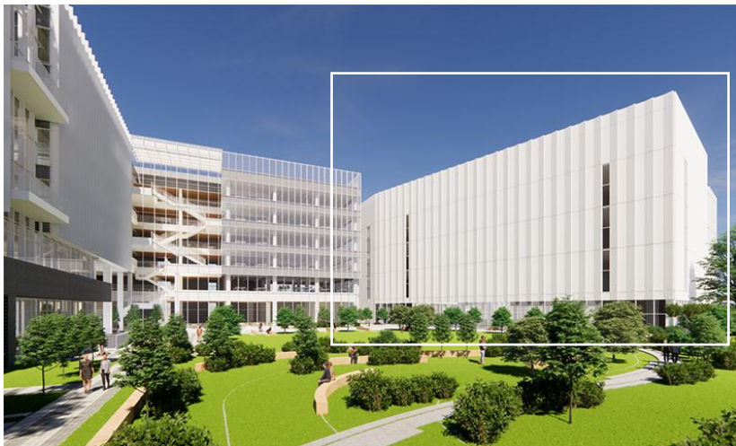
▲ Perspective View of the Gwacheon New Office Building and Data Center(In the Gwacheon Knowledge Information Town)
