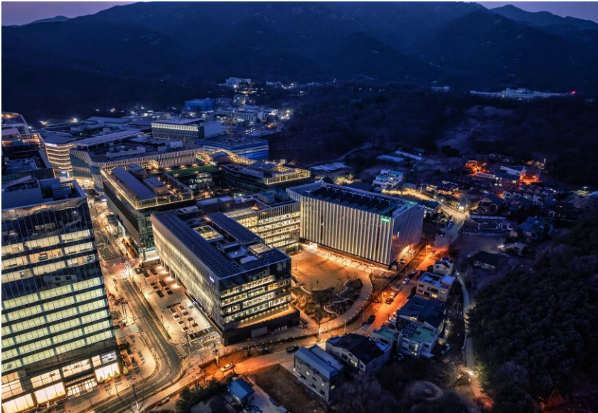
▲ Air view of the Gwacheon New Office Building and Data Center (In the Gwacheon Knowledge Information Town)
